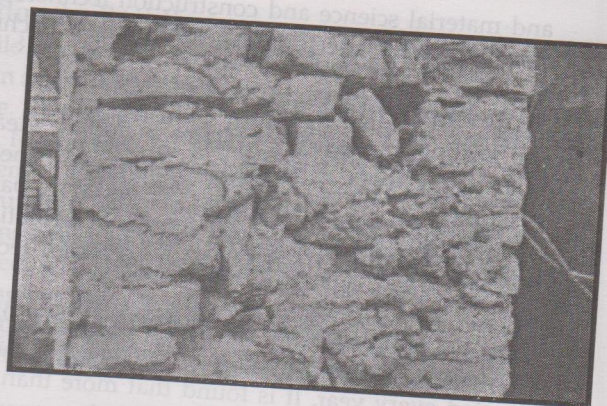
A typical traditional type of composite wall section.
