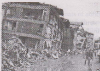
Fig.1. Collapse of buildings due to soft first storeys (1999 Turkey earthquake)
